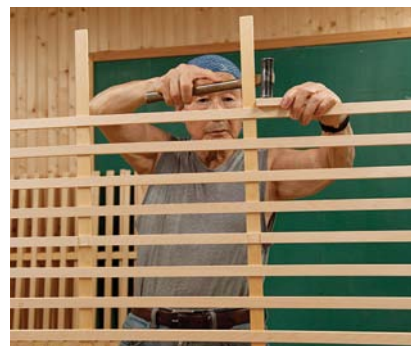
Coming through. The horizontal braces pass through mortises in the vertical lattice pieces.
