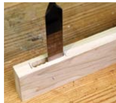
In the groove. Incisions from a marking gauge provide a place to locate the end of a wide chisel. When the chisel is in place, little effort is needed to shave off the high spots left by the drill bit.
