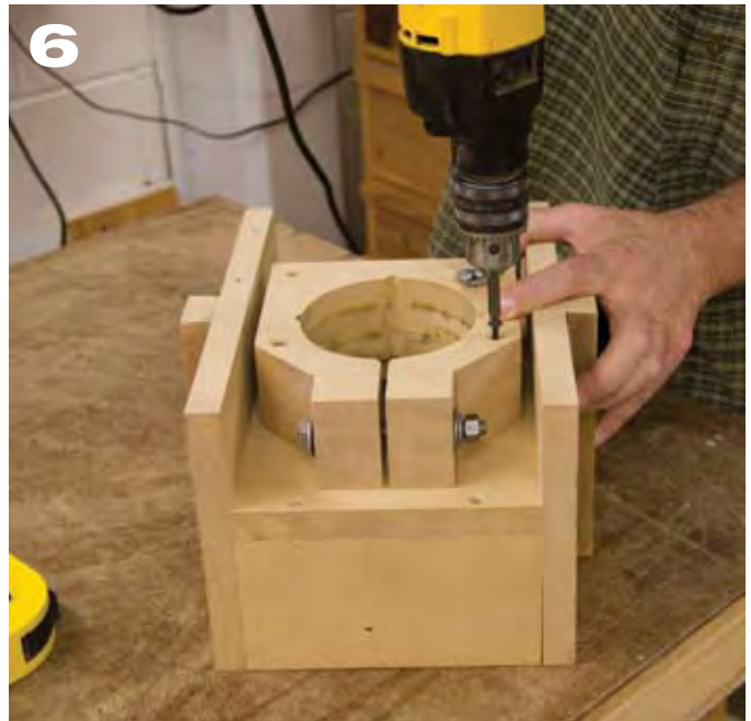
6 Attach the collar assembly to the carriage box, centering it over the oversized hole in the deck plate.
