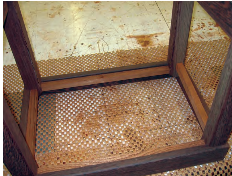
14 Cut spacers to fit snugly between the legs around all four sides of the inside of the apron. (These will hold the legs tightly in place against the corners during installation.) Apply glue to the two shoulder faces on each leg, set them into the corners and lock them snugly in place with the temporary spacers.
